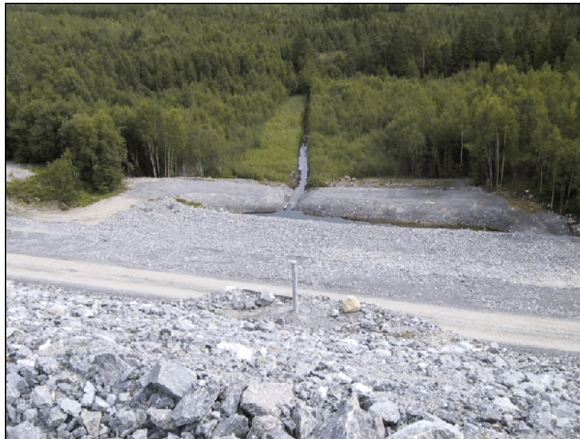
Figure 3.23: Another ditch for collection and flow measuring of seepage water alongside the dam [66, Base metals group, 2002]
