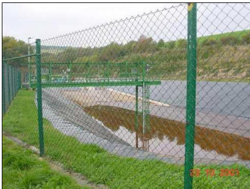
Figure 3.75: Water retention basin of German potash mine
