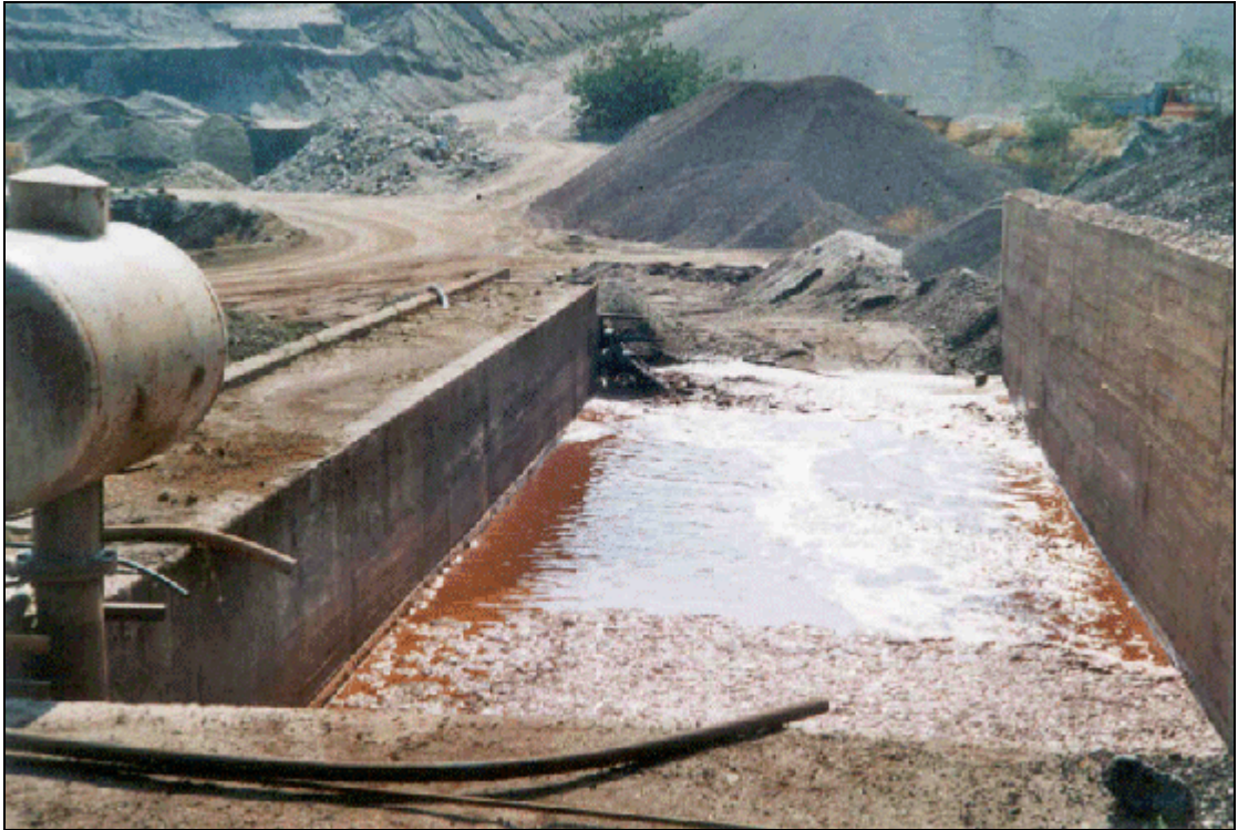
Figure 1.24: Example of a small tailings settling basin
